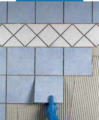
Installation of single-fired tile on gypsum board wall
