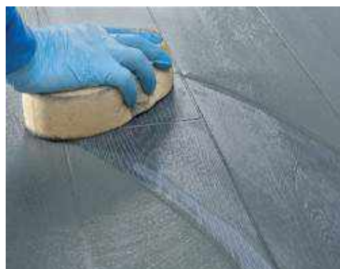
Cleaning and finishing the joints with a hard cellulose sponge
