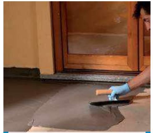
Waterproofing of terraces by trowel
