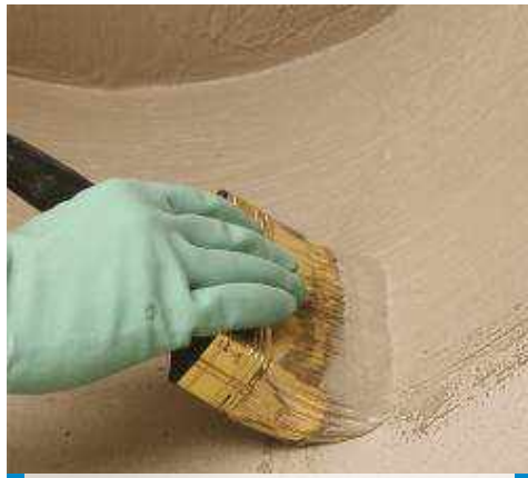
Waterproofing of details by brush
