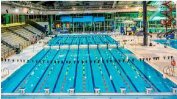
Completed 50 m pool at the Adelaide Aquatic Centre
