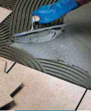
Installation of single-fired tile on floor
