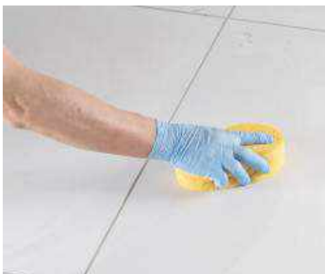
Cleaning and finishing the joints with a hard cellulose sponge
