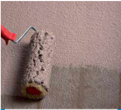
Waterproofing of details by roller
