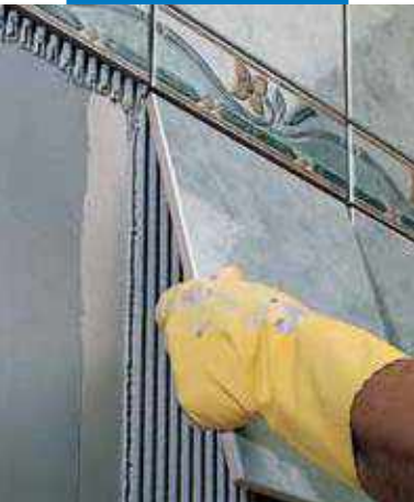
Installation of single-fired tile on wall render
